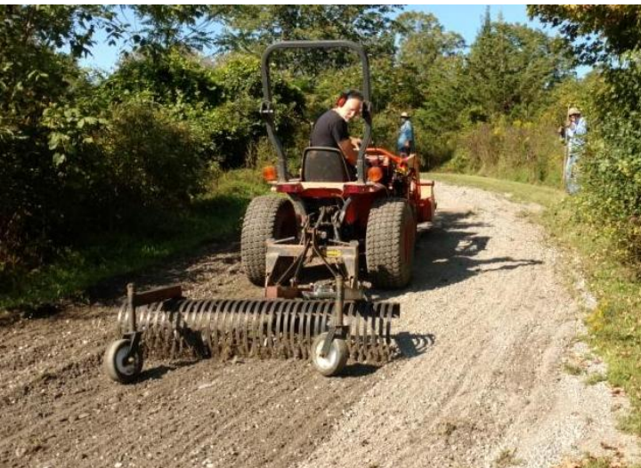
Repairing the driveway - AGAIN - after a bad rain-Oct 2
